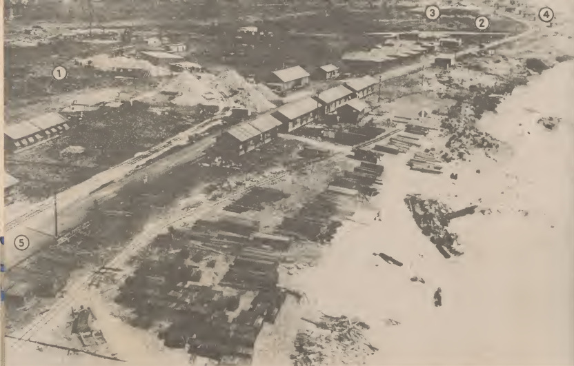
View due east from point near No. 1 Powerhouse. 1—Present Cracking Plant area. 2—Site of "Cat" Cracker. 3—Old Hospital, later Personnel Building, now site of "Cat Plant" Com-
